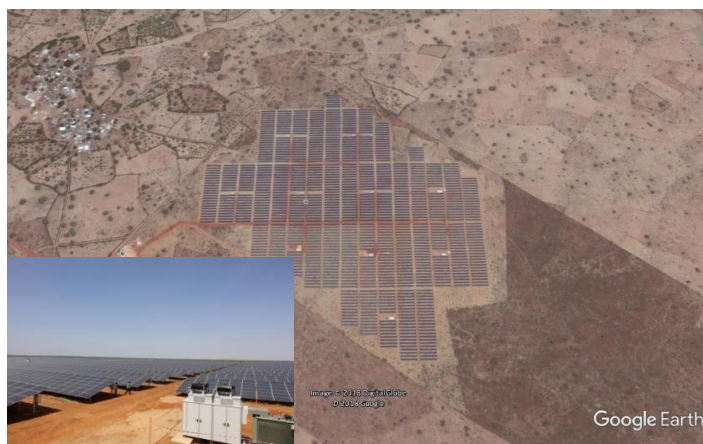
Malicounda 22 MW PV plant, Thiès region. Source: Google Earth
