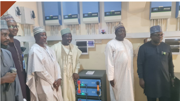
NIGERIA - Solar Power Installation at Bayero University, Kano
