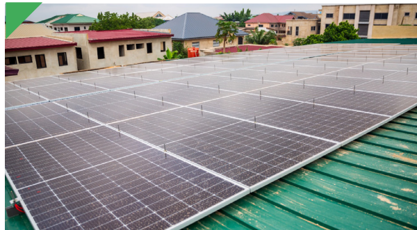
GHANA - 3 Hospitals benefited from Solar PV Installation
